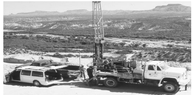
Standard Penetration Test (SPT)
